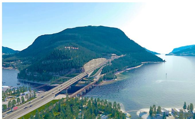
The Highway 1 four-laning project includes approximately 1.9 km of Highway, replacement of the existing R.W. Bruhn Bridge with a new four-lane bridge, and intersection improvements between Old Sicamous Road and Silver Sands Road.
